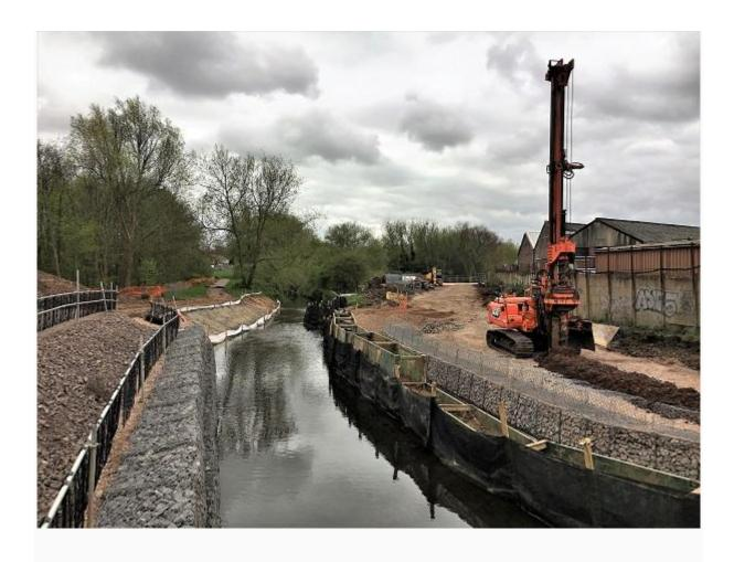
Image below: The eastern bund (flood defence embankment) is being constructed parallel with the rear of Ashbrook Road. The impermeable clay core of the bund is being laid on top of a clay foundation and will be packed down by a rolling machine. Sloping flanks will then be constructed on either side and the structure covered with topsoil and grassed over.
