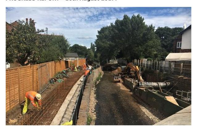
The image shows the view from Dogpool Bridge, looking downstream, where work has started on constructing the foundations of flood defence walls on both sides of the channel. The walls will rise to approx 1 metre above current bank top level and extend a few hundred metres downstream, protecting the properties on each side of the bank from being flooded by the river at times of extreme flow.
