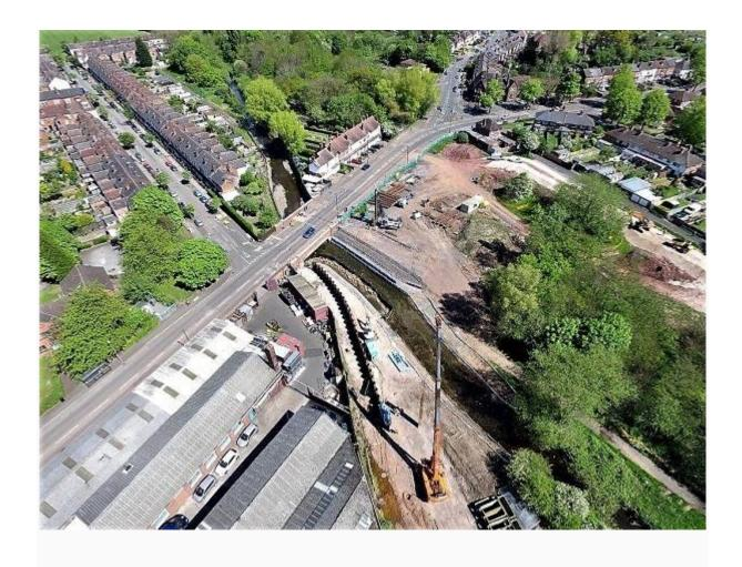
The UPPER IMAGE shows the site viewed from the south west. Dogpool Bridge is in the centre of the image and the sheet piling work on the western (left) bank is visible. Over to the right the recent construction work on the Ashbrtook Road bund is visible.
