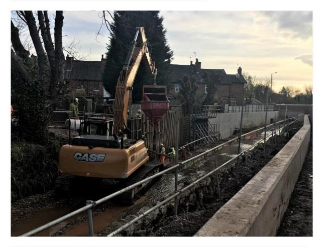
The image shows the view upstream towards Dogpool Bridge. The building of the flood defence wall on the Cecil Road side (right) has been completed as has much of the construction of the flood defence wall on the Moor Green Lane side (left). Work continues on the remaining section of this wall where concrete pouring is currently taking place.
