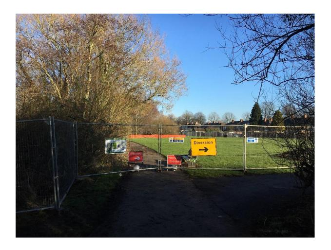
Preparation of the land within the fenced off area has continued. Low quality scrub vegetation has been cut down and scraped away and temporary plastic meshing fencing put around the more substantial clumps of trees which will remain. Marker stakes have been put in position indicating the line which the bund will follow.
