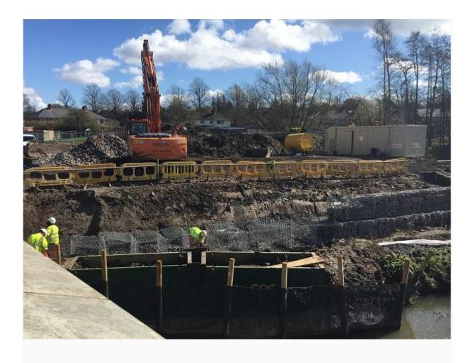
Meanwhile, running parallel behind the houses in Ashbrook Road the foundations for a bund (flood defence embankment) are being created by infilling the previously excavated trench with impermeable clay. This prevents water from forcing its way under the bund.
