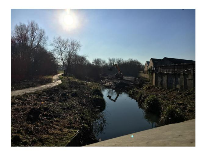
In the coming weeks, work will begin on diverting the river as seem in this last image a short distance eastwards (to the left) to create a wider area of land on the western bank (on the right of the picture) for the building of the flood defence wall. Daytime traffic signals will operative outside peaks times to allow the creation of a temporary access route for heavy machinery across the west bank parkland. The parkland will be fully restored in the final stages of the project
