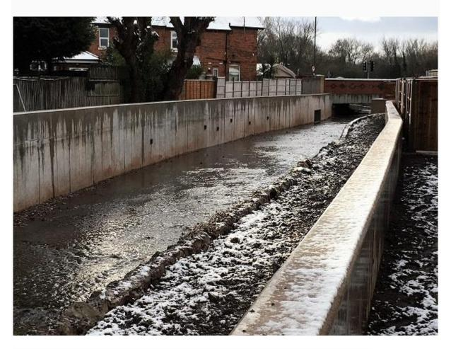
The image shows part of the Selly Park South Flood Risk Management Scheme (FRMS), viewed upstream towards Dogpool Bridge. The building of flood defence walls between the rear of Cecil Road and Moor Green Lane is now completed which marks the end of the main construction phase of the FRMS, meaning that the scheme is fully operational reducing the risk of river
