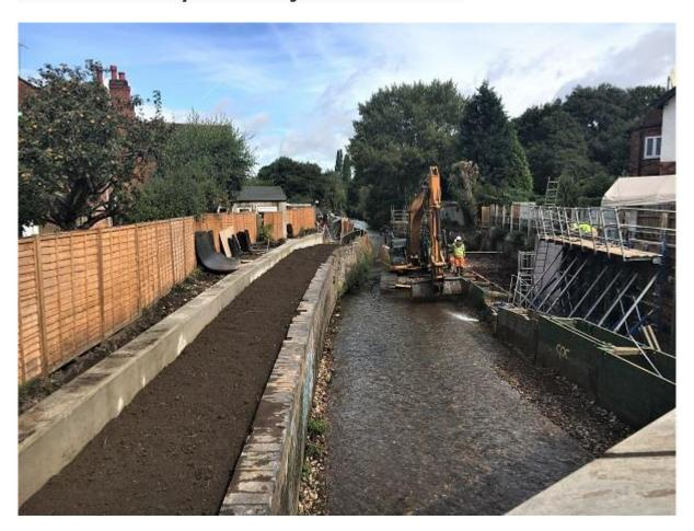
The image above shows the view from Dogpool Bridge, looking downstream, where work is now well underway constructing flood defence walls on both sides of the channel. The walls will rise to approx 1 metre above current bank top level and extend a few hundred metres downstream, protecting the properties on each side of the bank from being flooded by the river at times of extreme flow.
