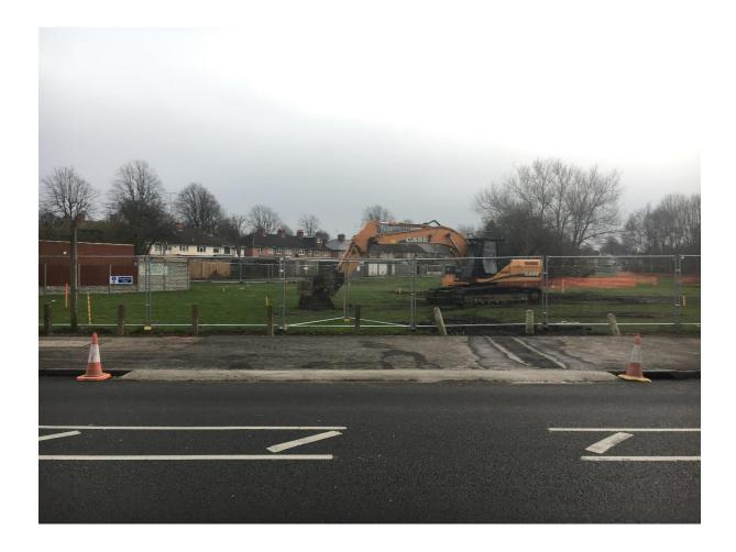
PROGRESS REPORT Friday 3rd February - Work ongoing during the FIRST week of FEBRUARY: Extensive preparation of the land on the east side of the river by heavy machinery for construction of the flood protection bund which will run alongside Moor Green Lane and along the back of Ashbrook Road. The parkland will be fully restored in the final stages of the project.
