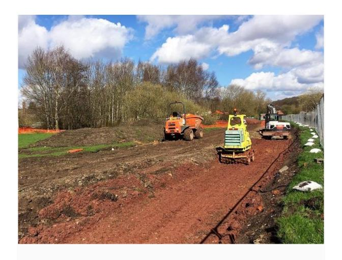
PROGRESS REPORT Thursday 13th April - Work ongoing during the SECOND and THIRD week of APRIL: Image below: Work is almost complete on diverting the channel of the River Rea just upstream from Dogpool Bridge. The channel has been moved a short distance to the east to allow access for heavy machinery to construct the flood defence wall on the western side of the river. The drilling machine is preparing the ground along the line where the concrete slabs of the wall will be piled into the ground.
