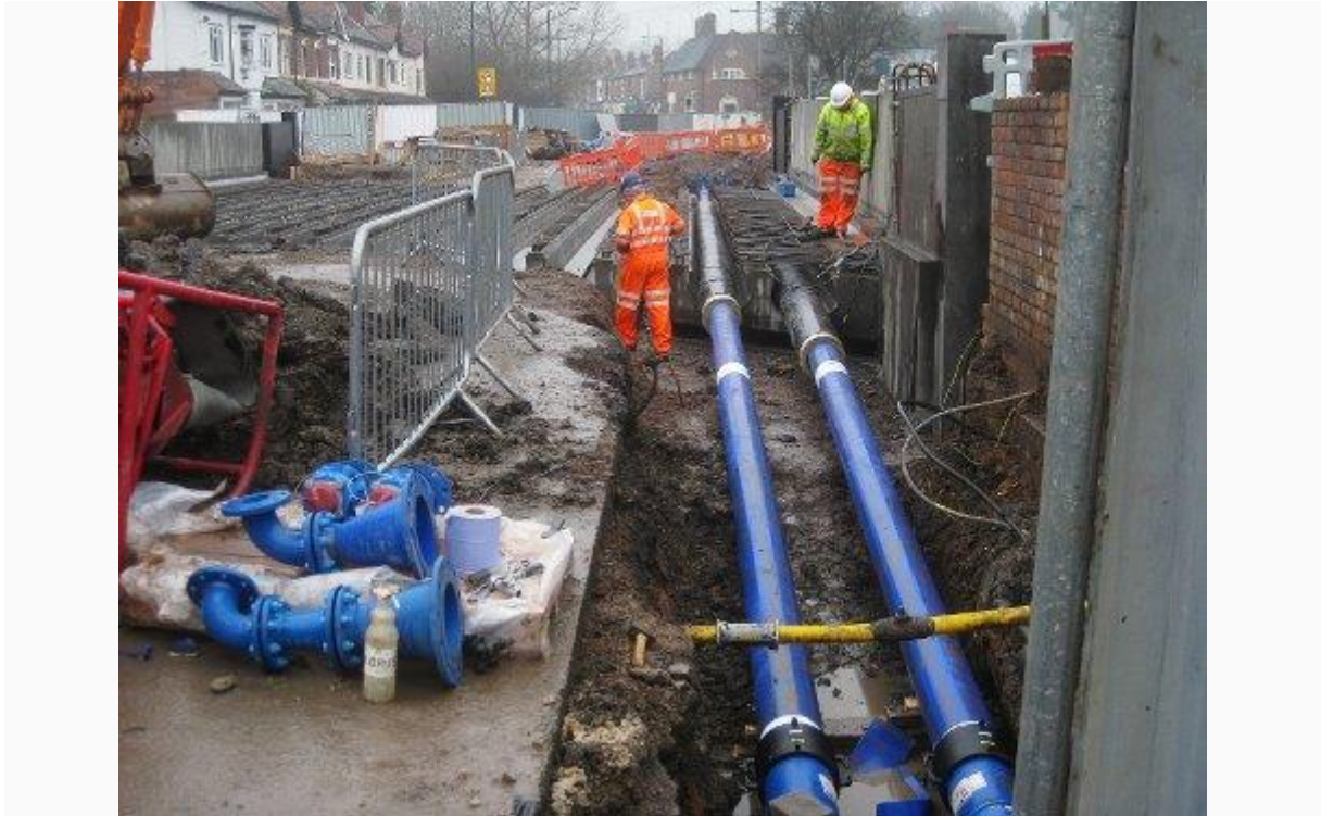
Image above: Thursday 7th March - Severn Trent water mains being installed across the new bridge.
