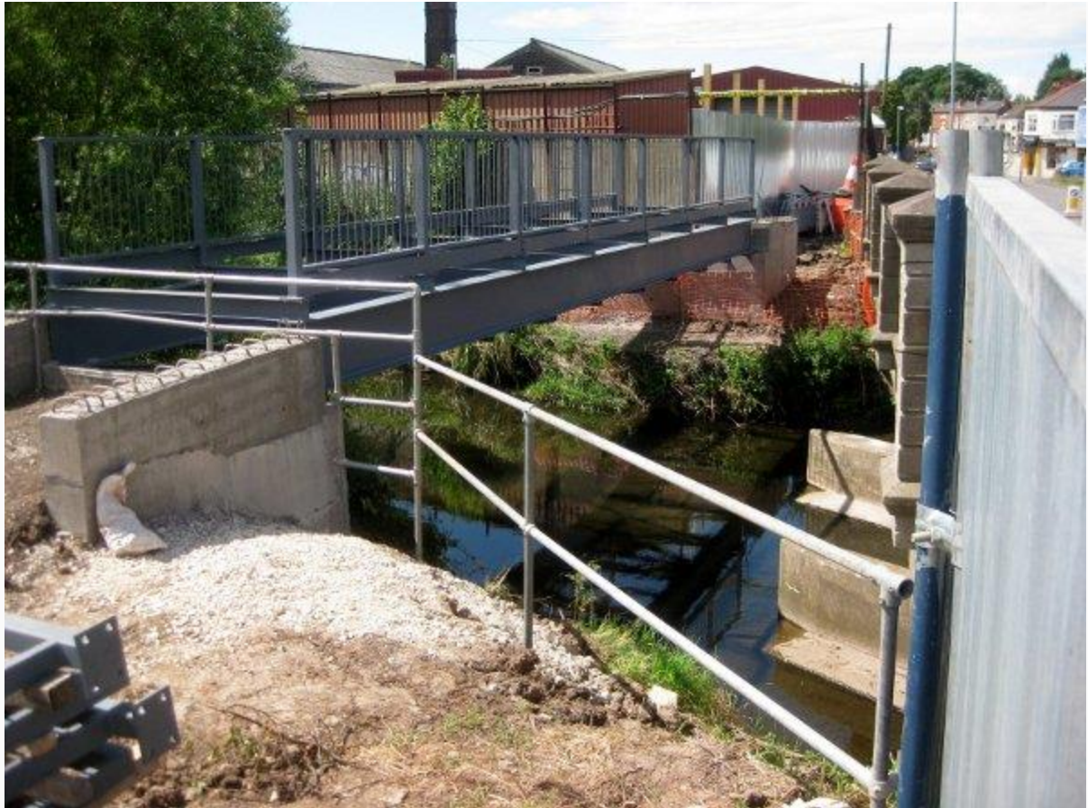
Above: The steel frame of the temporary bridge in place alongside the road bridge.
