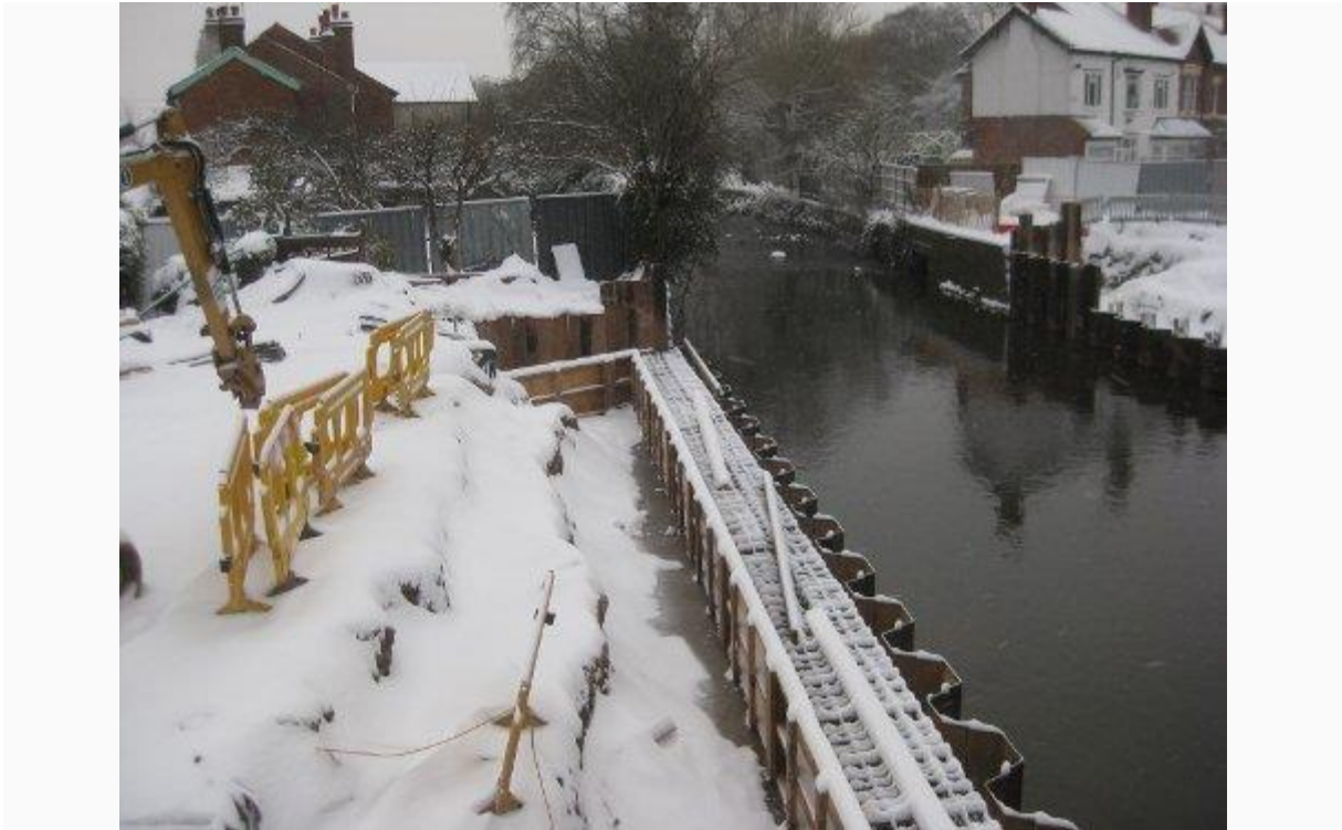
Image above: Preparatory work for concrete casting on the western (Dogpool Lane) bank of the river.
